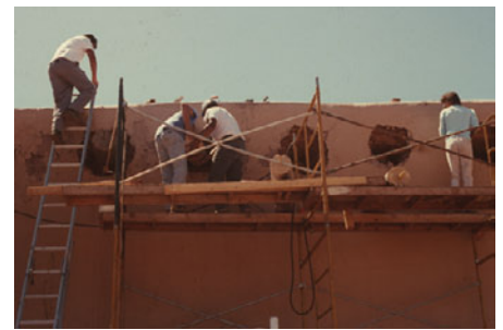
New viga ends were screwed into place.
