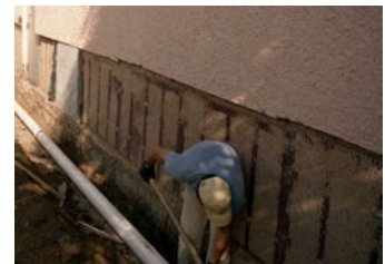
Cages supporting a failing wall at Zia Diner, Santa Fe.
