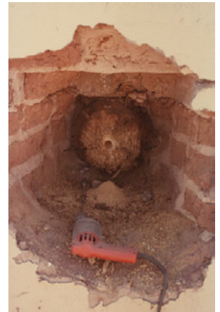
Viga was prepared for splice.
