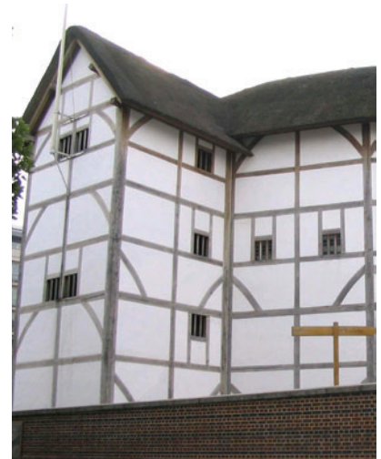
Exterior lime plaster at the Globe Theatre reconstruction.
