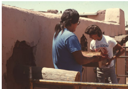
Viga end was removed.
