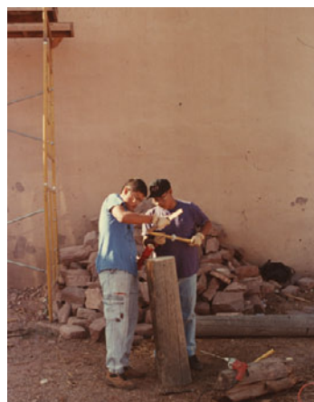
A threaded fiberglass rod was installed in the new tail.
