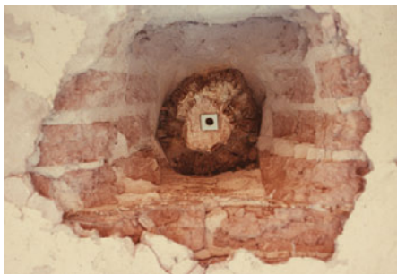
Fiberglass nut was epoxied into place.
