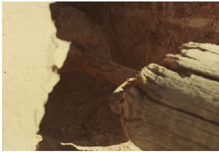
Rotted viga ends were discovered.
