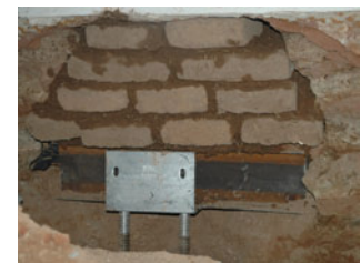
Helical pier supports basket at reconstructed adobe wall base.
