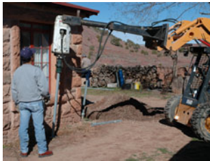
Helical pier installation, Hubbell Trading Post National Historic Site.
