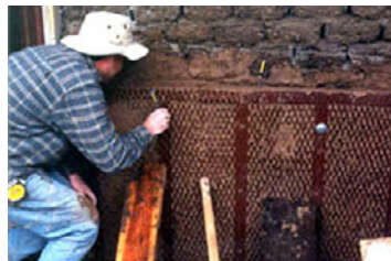
Installation of cages, historic Seco Plaza Complex, Arroyo Seco.
