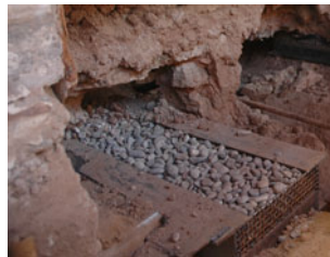
Basket in place under a failed wall, historic home, Bernalillo.
