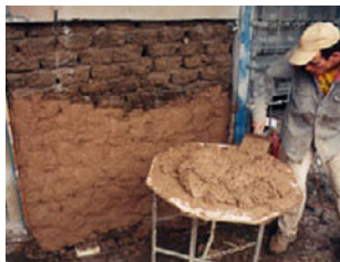
A lime-rich mud is cast onto the damaged adobe wall.
